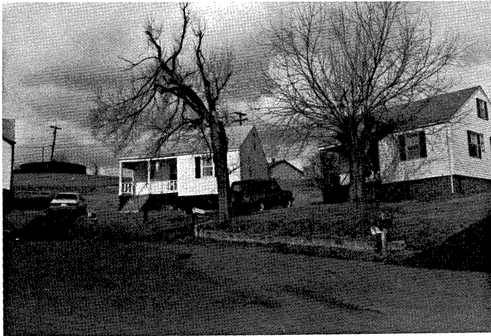
Plate 15. Houses at Victory Heights, Christiansburg, Virginia, February 1995.
